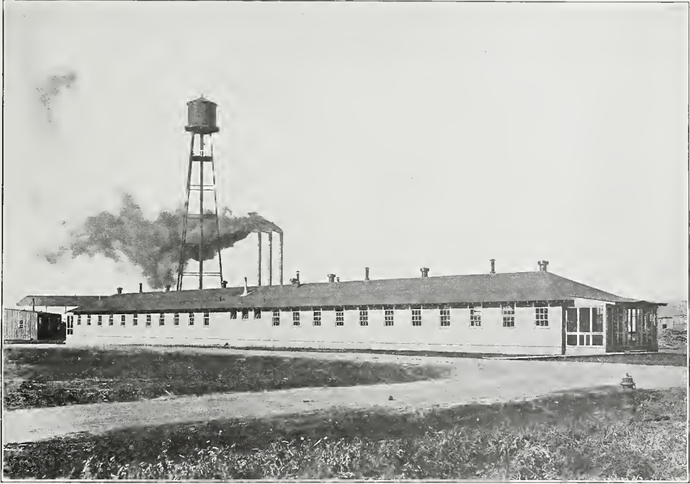
FIG. 129.—Enlisted men's barracks, Post Hospital, Wilbur Wright Field, Ohio.
